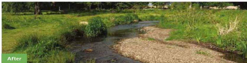
Figure 2.27. The Braid Burn, Edinburgh, before and one year after work to lower an artificial raised bank and replace the concrete channel with sinuous meanders: This work formed part of wider flood alleviation works carried out by the City of Edinburgh Council that sought to also improve biodiversity and public amenity on this watercourse (© River Restoration Centre).
